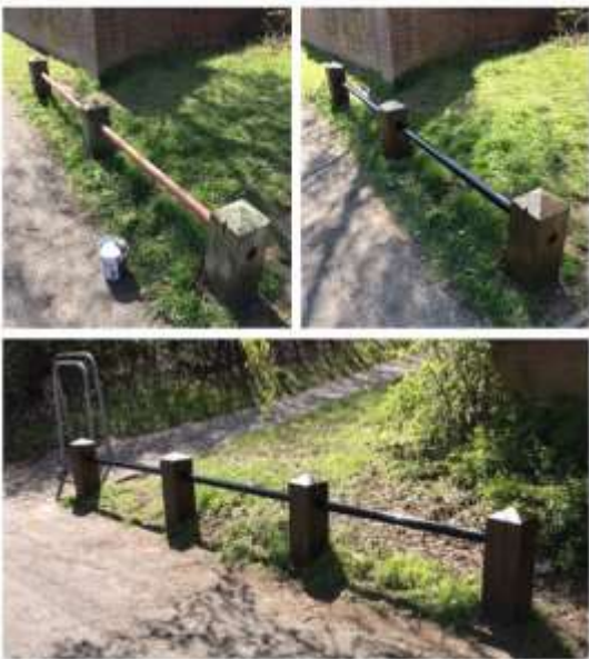
Barriers painted and posts stained.
