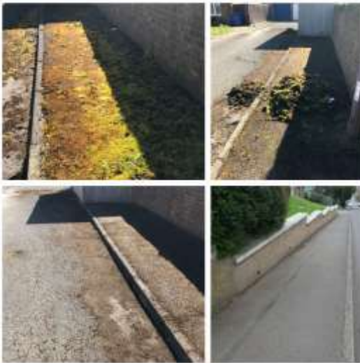
Cleared moss from path on John Street.
