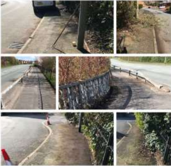
Cleared paths on Brickworks Road.
