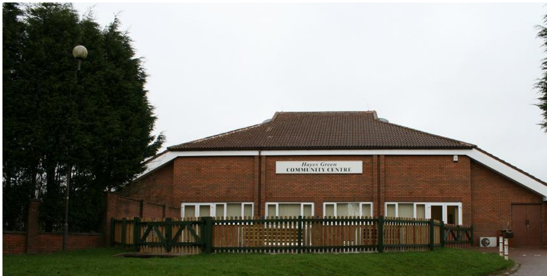
Hayes Green Community Centre, rear view above and internal below.
